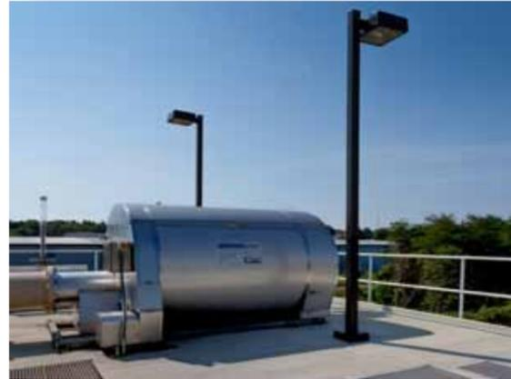
Mechanical Drum Screen at Headworks
